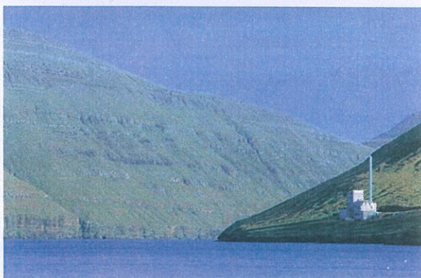
Waste-to-energy plant in Leirvik, Faroe Islands Client: IRF Architect: Køhler & Jørgensen
