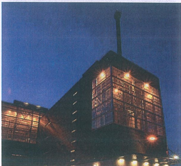
Waste-to-energy plant in Halmstad, Sweden Client: RenhållningsBolaget Architect: Liljewall Arkitekter AB
