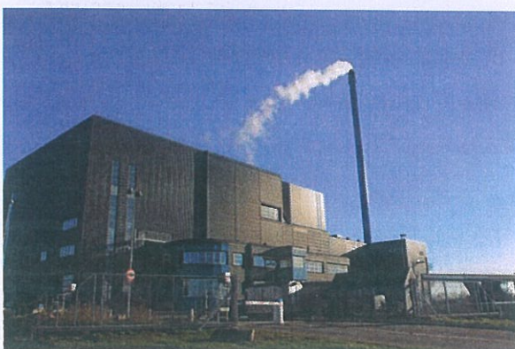
Waste-to-energy plant in Hjørring, Denmark Client: I/S AVV Architect: Finn Østergaards Tegnastue
