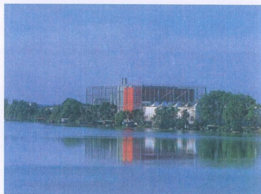
Waste-to-energy plant in Bordeaux, France Note the low stack height
